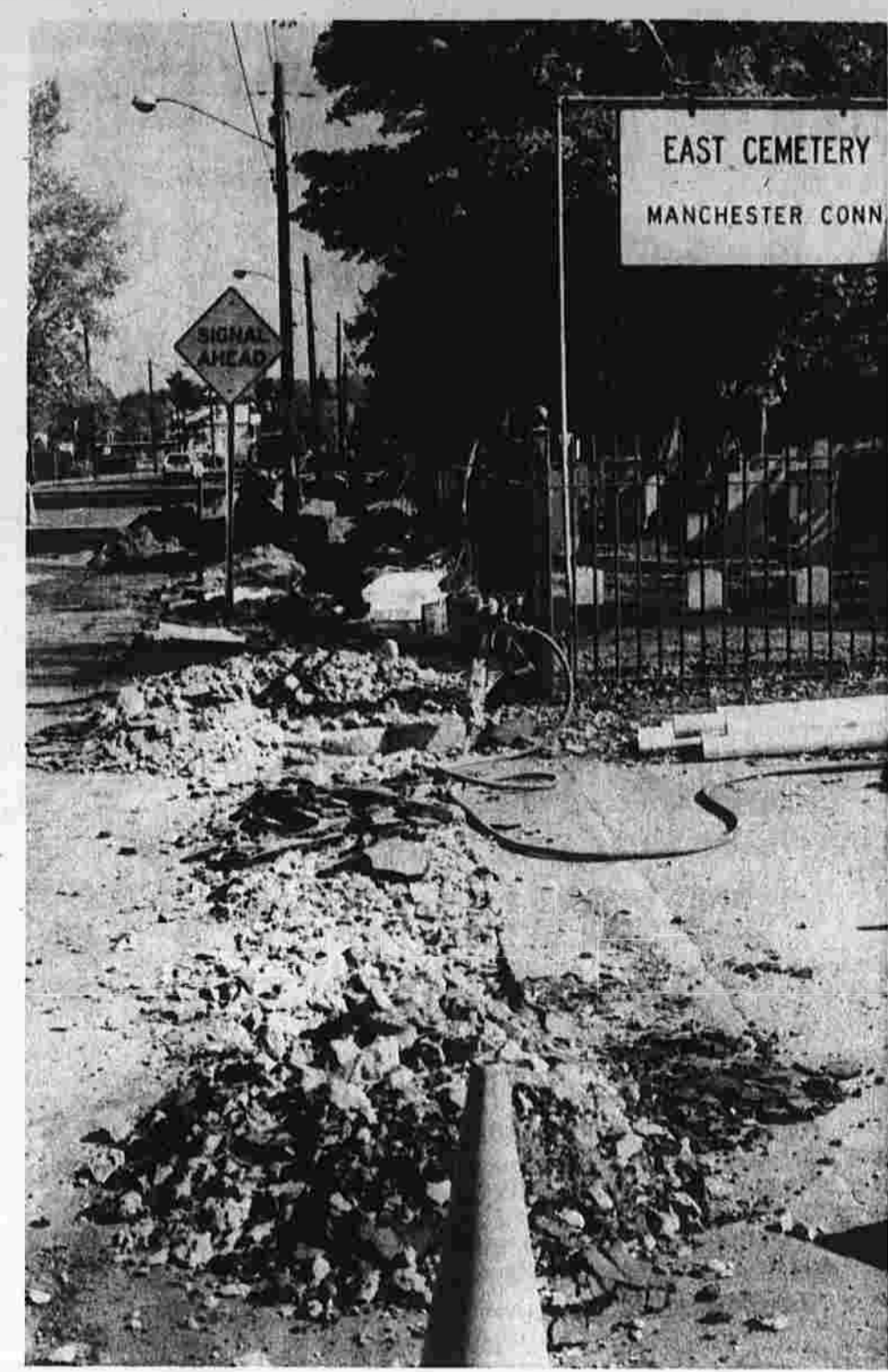
SNET Lines Go Underground
